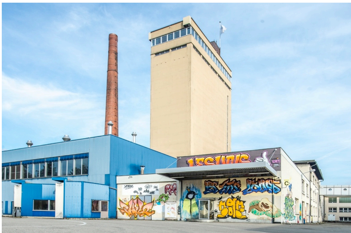
blueFACTORY, Fribourg. Photo : Adrian Moser
